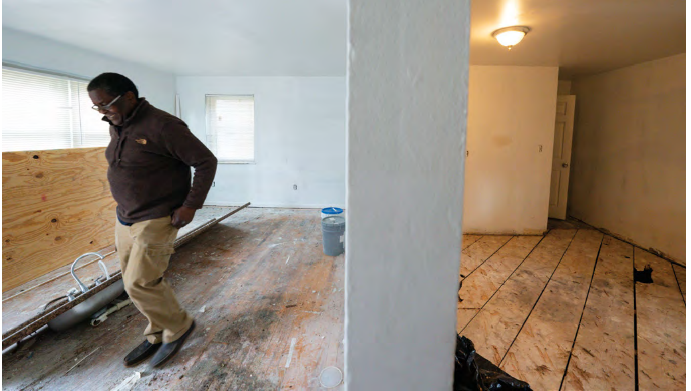
A contractor hired by the Port examines the condition of one of the agency's newly purchased houses. Credit: Jeff Dean.
