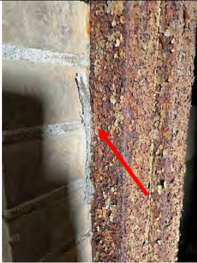
Photo 2 HA 22: Asbestos-Containing Gray Interior Door Caulking
