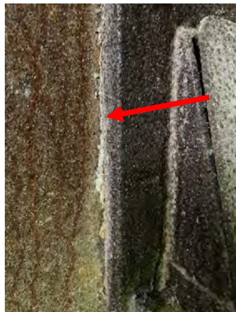
Photo 5 HA 26: Asbestos-Containing White Gasket Material
