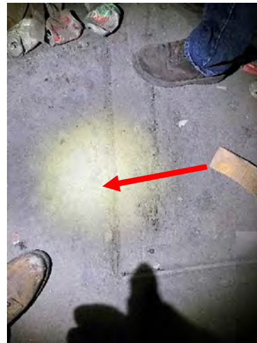
Photo 4 HA 25: Asbestos-Containing Black Tar
