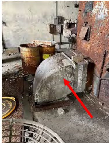
Photo 21: Asbestos-Containing Cementitious Insulation and Wire Mesh
