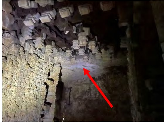
Photo 26: Asbestos-Containing Trowel-Applied Fibrous Insulation
