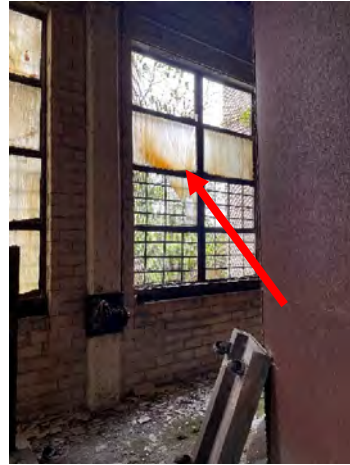
Photo 8 HA 29: Asbestos-Containing White Exterior Window Glazing
