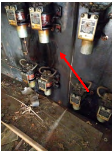
Photo 11 HA 33: Asbestos-Containing Black Backer Board
