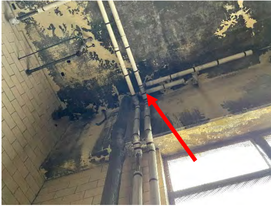
Photo 19: Asbestos-Containing Air-Cell Pipe Insulation and Mudded Fittings
