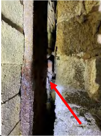
Photo 25: Asbestos-Containing Mineral/Glass Wool Insulation
