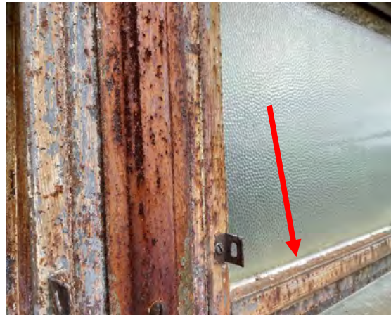
Photo 2 HA 23: Asbestos-Containing White Interior Window Glazing
