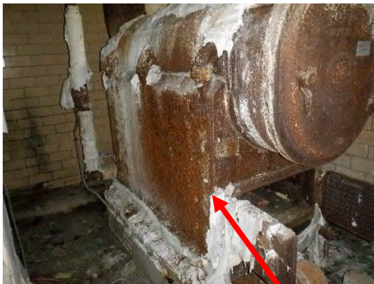
Photo 21: Asbestos-Containing Cementitious Insulation and Wire Mesh
