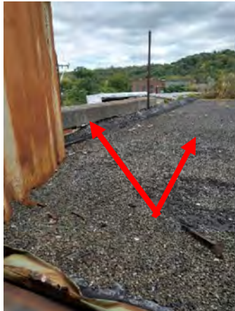
Photo 9 HA 30/31: Asbestos-Containing Tar Paper in the Built-Up Tar Roof System and Asbestos-Containing Flashing
