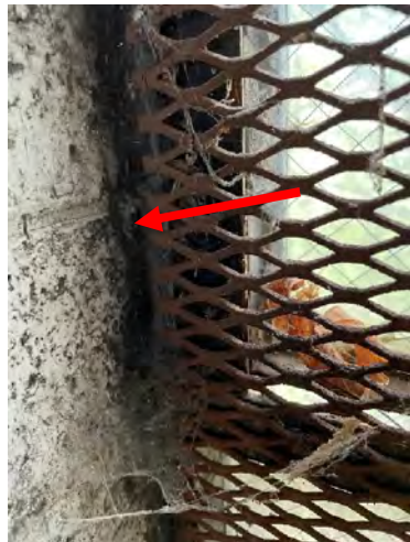
Photo 3 HA 24: Asbestos-Containing Gray Interior Window Caulking
