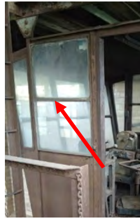
Photo 10 HA 32: Asbestos-Containing White Interior Window Glazing
