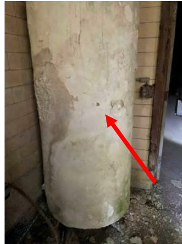
Photo 22: Asbestos-Containing Preformed Block Insulation
