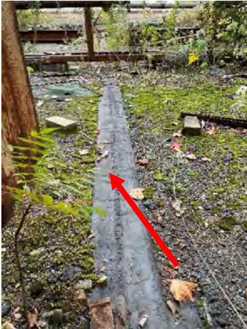
Photo 27: Asbestos-Containing Asphalt-Based Roofing Membrane
