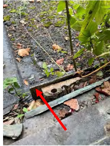
Photo 28: Asbestos-Containing Transite Panels
