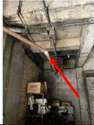
Photo 20: Asbestos-Containing Cementitious Pipe Fitting Insulation on Fiberglass Insulated Lines
