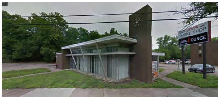
FORMER PROVIDENT BANK 1954 | 11173 READING ROAD | SHARONVILLE
