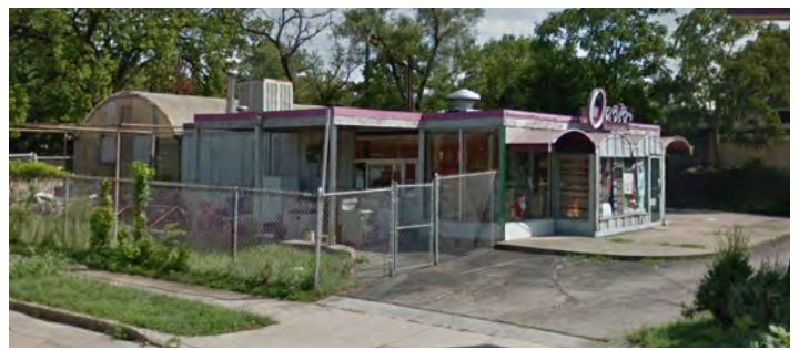
FORMER OASIS FLORIST 1963 | 9188 READING ROAD | READING
