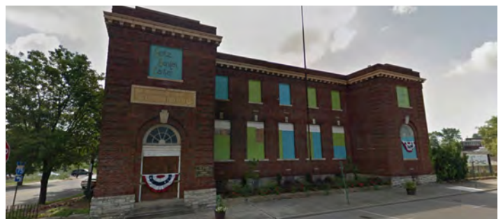
STEARNS & FOSTER OFFICES 200 E. WYOMING AVENUE | LOCKLAND
