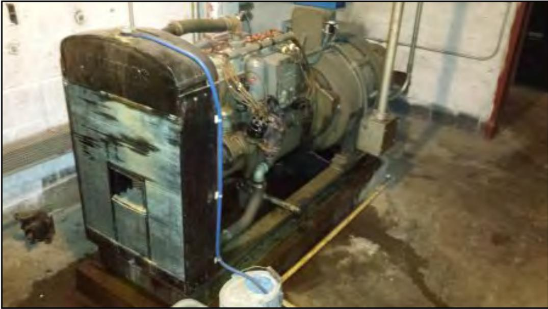
Generator motor. Note oil pan and staining.
