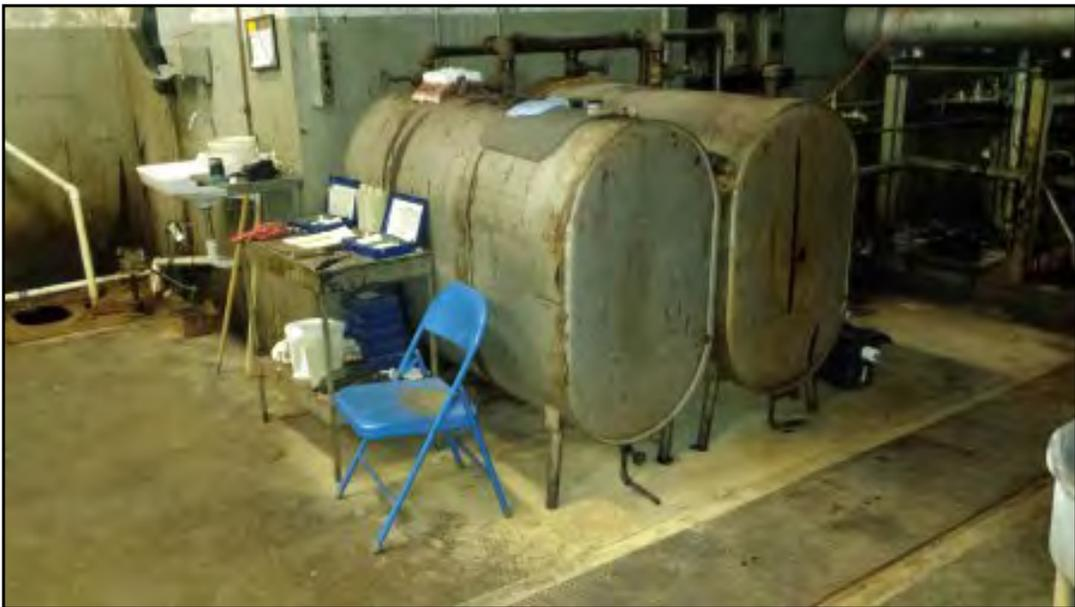
Heating oil ASTs formerly used to supply fuel to boilers.
