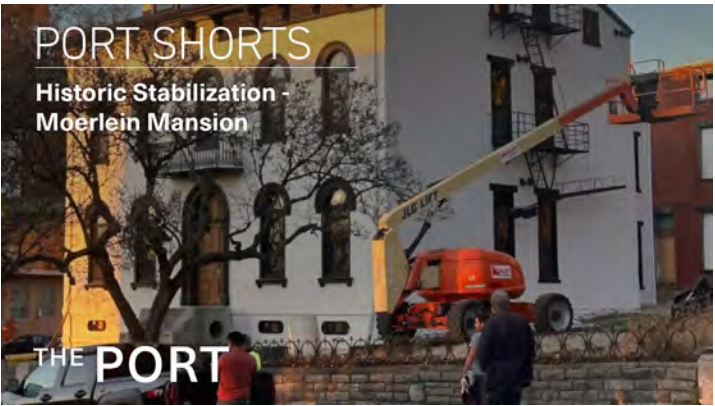
Historic Stabilization: Moerlein Mansion | June 2024
