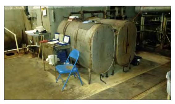
Heating oil ASTs formerly used to supply fuel to boilers.
