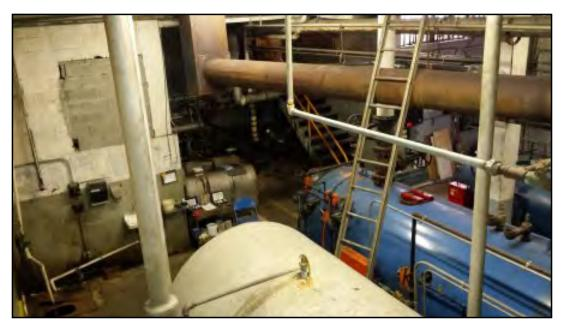
Boiler room. Note two fuel oil ASTs and three boiler tanks.
