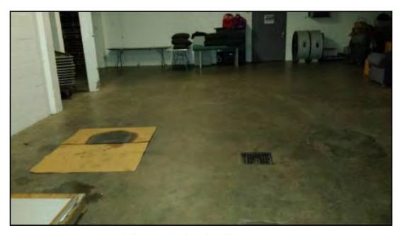
Hydraulic oil floor staining from forklifts in eastern storage area.
