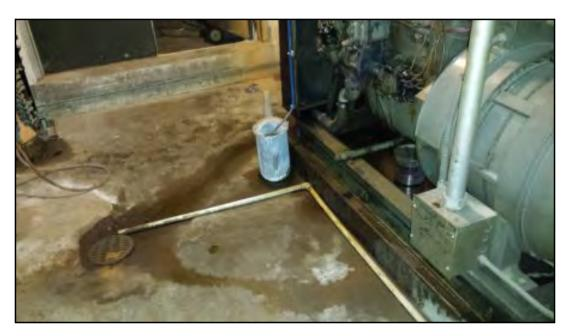
Generator motor and oil staining running to floor drain.
