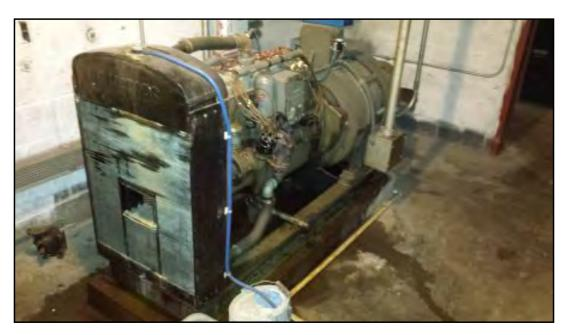
Generator motor. Note oil pan and staining.
