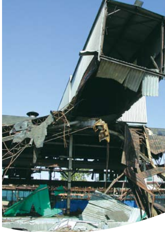
Building demolition at 3603 East Kemper Road
