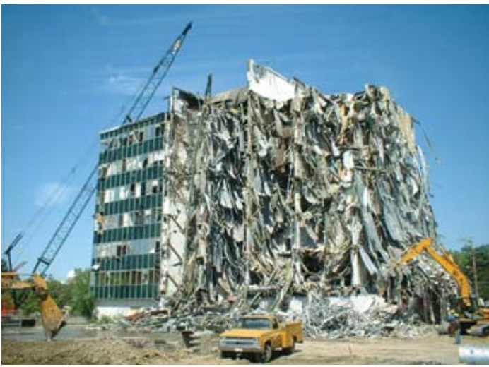
3333 Vine Street Project building demolition
