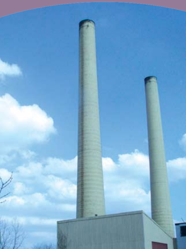
Incinerator at Center Hill Landfill
